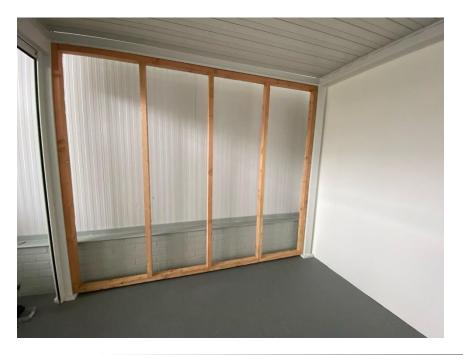
Step 3: After you have made the frame in the canopy, you can attach the boards to it. Start from the top. Drill the wooden boards to the frame. The top board should be level with the top of the rain gutter.
